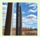
Steel H pilings installed to support D Street walls
